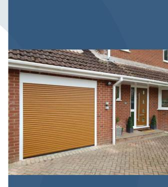
Contrasting guides and box for these doors fitted within the opening coordinate with other finishes.
